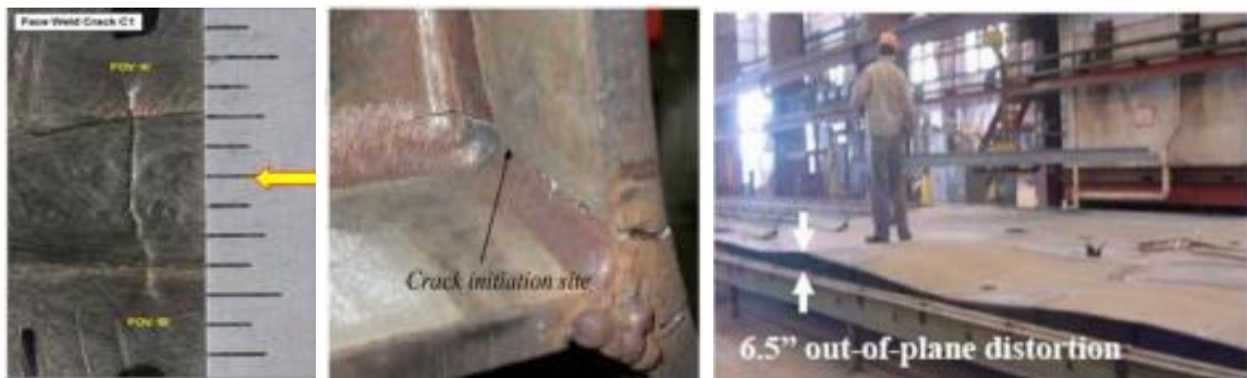
Figure 1: (a) Transverse crack in Titanium due to butt welding, (b) Corner cracks in FPSO unit (Song, 2012), (c) Large buckling distortion (Huang et al., 2007). These figures illustrate that the complex and Multiphysics nature of welding generated issues: residual stress and distortion can lead to severe issues and may result in catastrophic failure of the structure.
