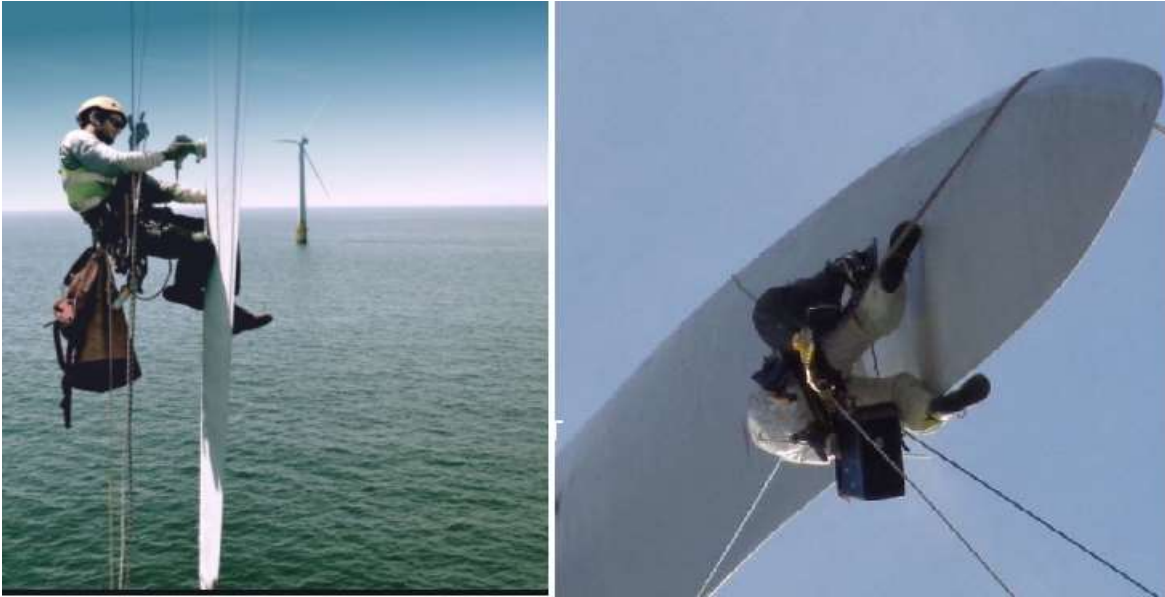
Figure 26: Blade repair offshore Source: https://www.altitec.co.uk/services
