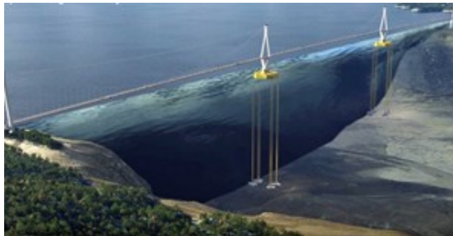
Figure 1.3: TLP-supported floating bridge on the Bjørnafjord crossing
