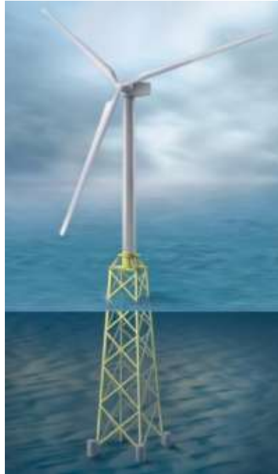
Figure 10 Jacket foundation (public domain).
