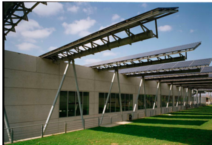
Figure 35. Protruding "wing" PV structures in the Rainbow Headquarters in Loreto, Italy (Scognamiglio & Røstvik, 2012, p. 12).
