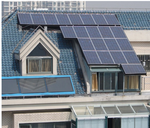
Figure 1-1 An example of a BAPV system [2]
