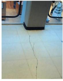
Figure 2-21 Cracking in tiles [23]
