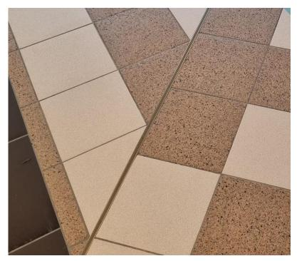
Figure 2-25 Movement joint in a local shopping mall.
