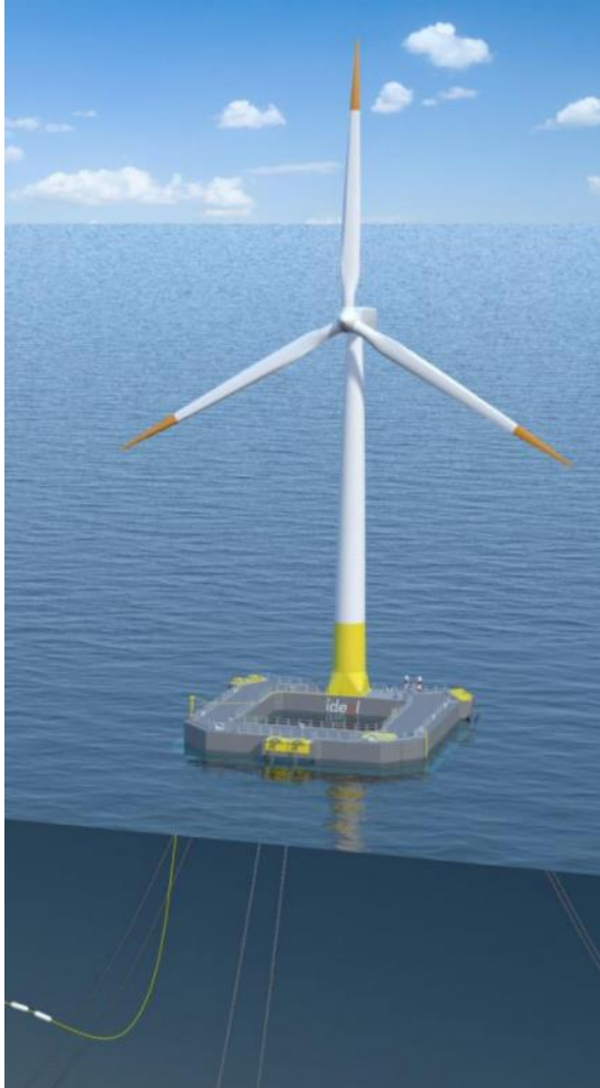
Figure 3.2 - BW Ideol's patented damping pool technology in use on a floating wind turbine[31]
