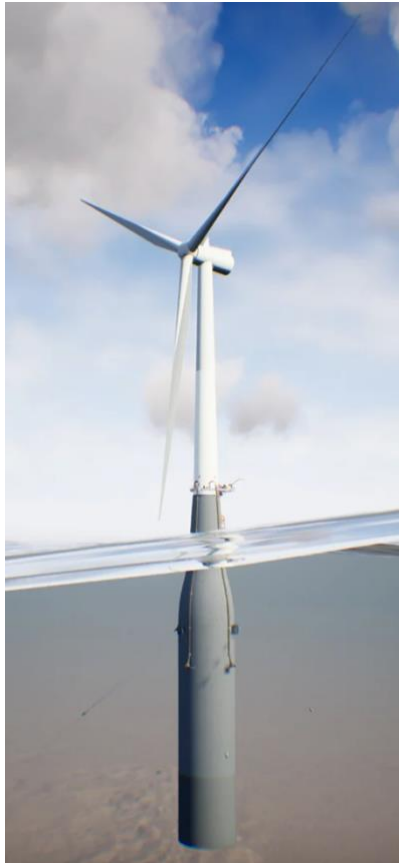
Figure 3.3 - Equinor's Hywind structure which utilizes SPAR buoy[33]
