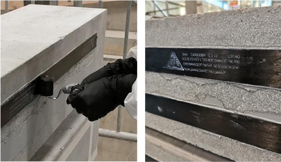
Figure 3.31 Bonding of the plates onto concrete substrate
