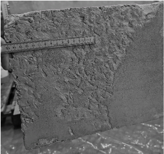
Figure 3.18 Beam A.3 after repair
