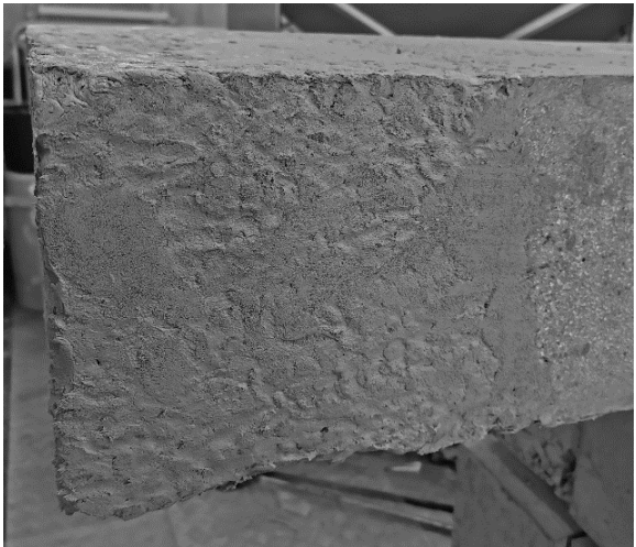
Figure 3.20 Beam A.4 after repair
