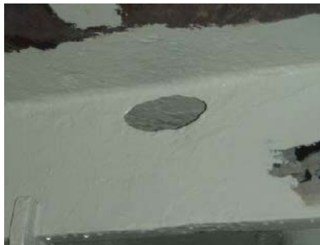
Picture 42 Maintained drain hole (Clipper Skagen 2009)
