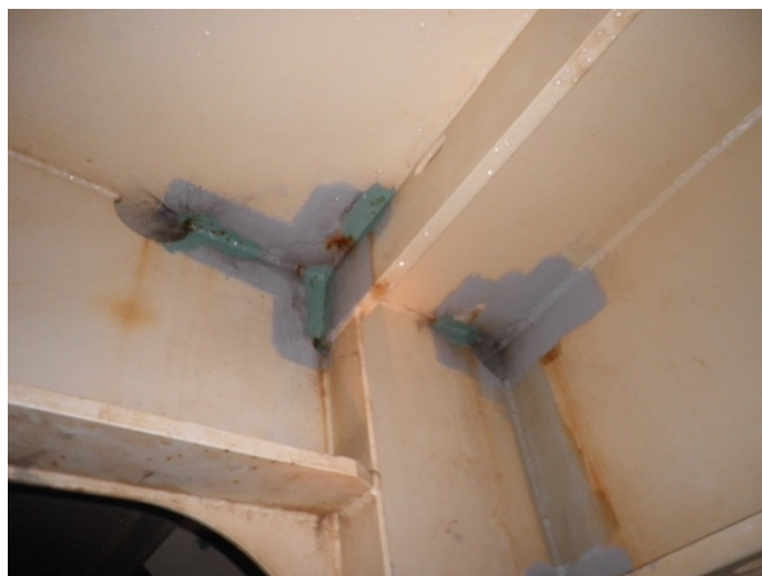
Picture 66 Deckhead (Ask 2014b)
