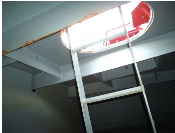
Picture 76 Corrosion on longitudinal near manhole (Clipper Mars 2013)
