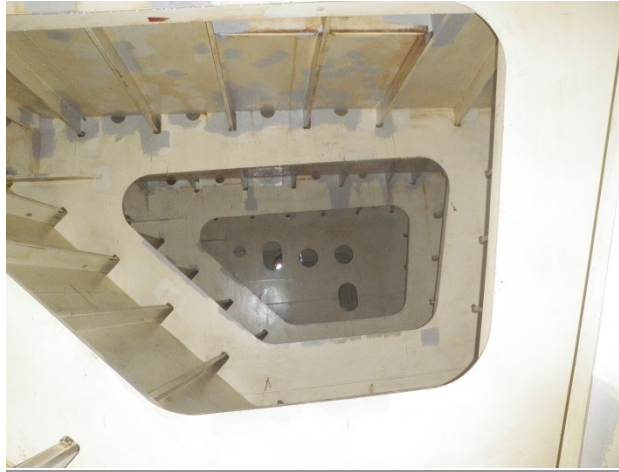
Picture 60 General condition wing ballast tank (Clipper Harald 2012a)
