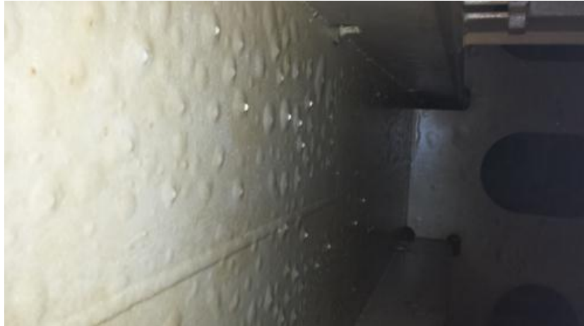
Picture 26 Blisters in the ballast tank in Clipper Skagen (Solvang 2012)
