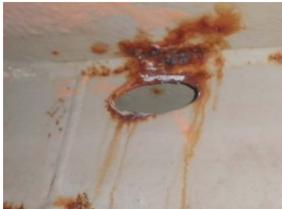
Picture 12 Edge breakdown in drain hole (Ask 2014a)
