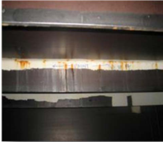
Picture 71 Corrosion on weld seams in deckhead (Clipper Star 2014)
