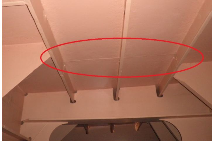
Picture 94 Butt-weld in deck-plating (Skagen 2014)
