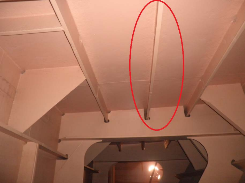
Picture 2 Longitudinal under deck plating
