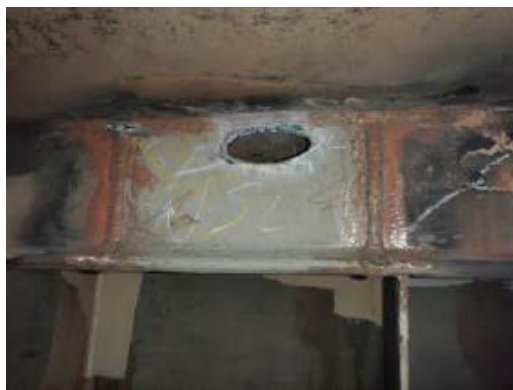
Picture 43 Renewed drain hole (Clipper Skagen 2009)
