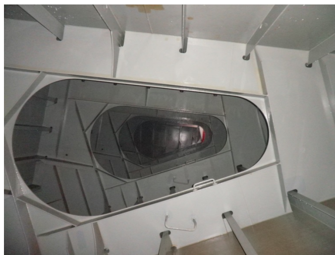
Picture 87 General condition of wing ballast tanks (Ask 2014c)
