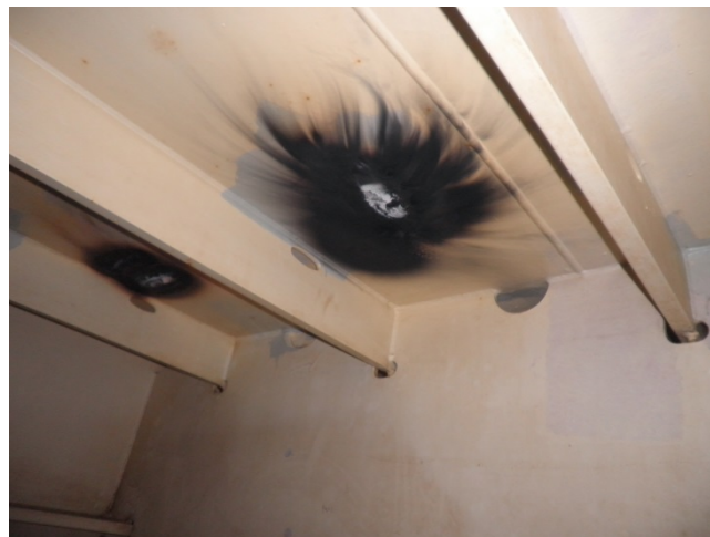
Picture 68 Deckhead after welding on deck (Ask 2014b)
