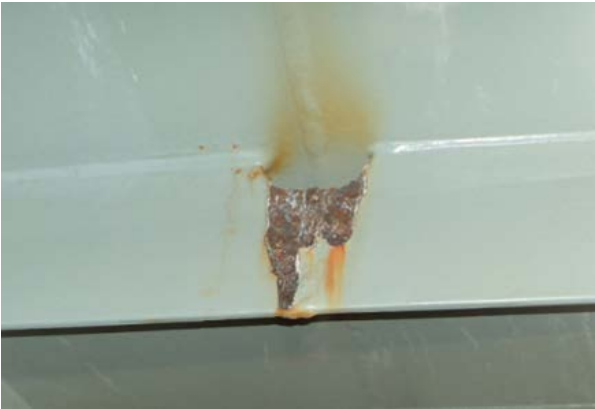
Picture 18 Drain hole in a wing ballast tank (Clipper Mars 2014)
