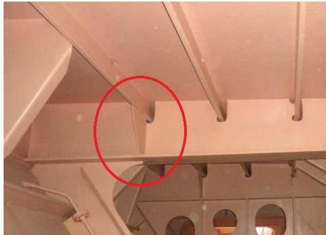
Picture 93 Stiffener support in top of wing ballast tank (Skagen 2014)
