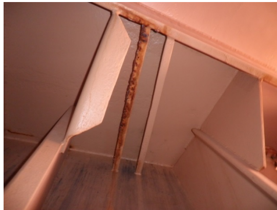
Picture 57 Two years after recoating (Ask 2014a)
