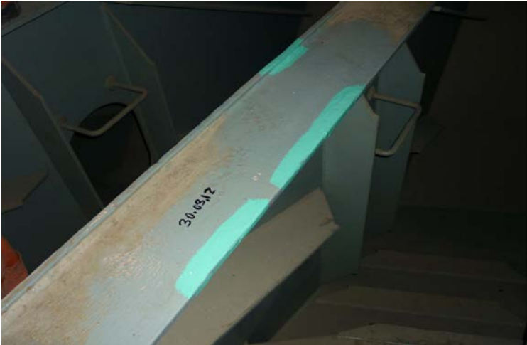
Picture 31 Corrosion repair with date (Solvang 2012)
