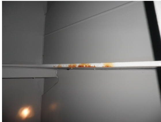
Picture 11 Edge breakdown on Clipper Posh (Ask 2014c)
