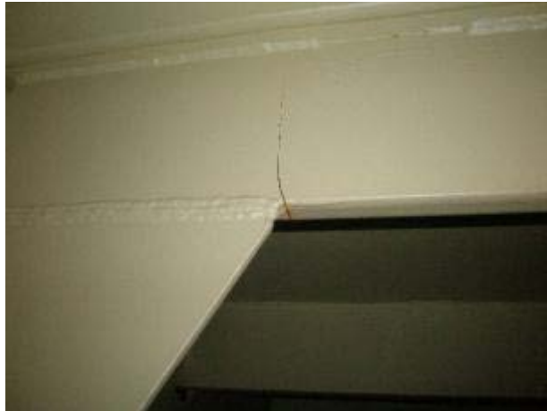
Picture 7 Crack on a high stress concentration area (Clipper Skagen 2012)
