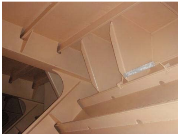
Picture 53 After grit blasting and recoating (Clipper Skagen 2012)
