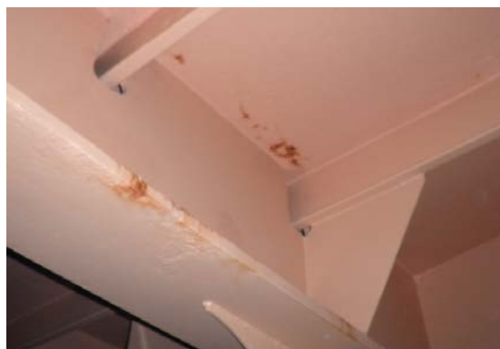
Picture 58 Two years after recoating (Ask 2014a)
