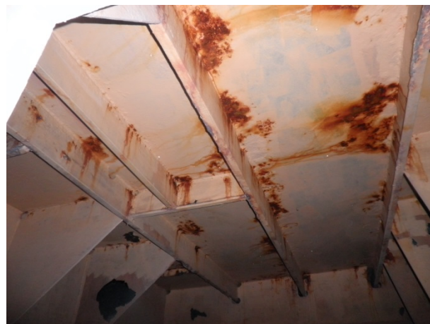
Picture 21 Top of a wing ballast tank (Ask 2014a)
