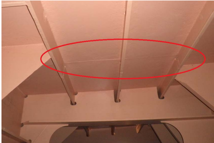
Picture 4 Butt-weld in deck plating
