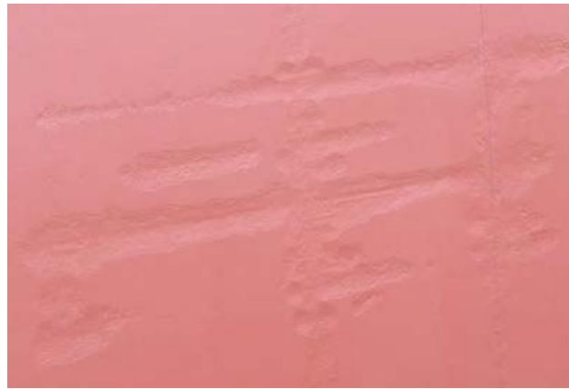
Picture 4 Grooving corrosion on ship's side after grit blasting and coating (Clipper Victory 2013)
