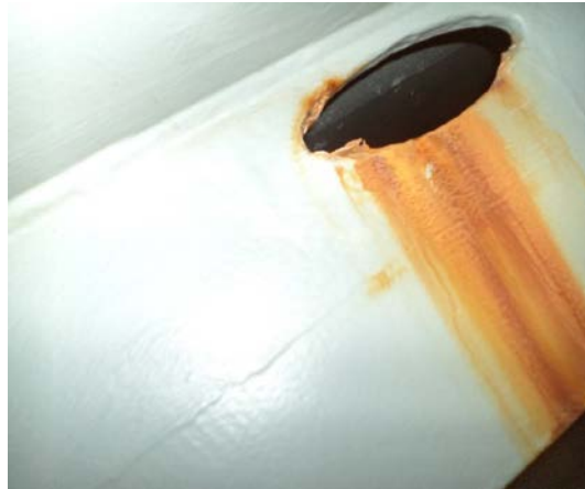
Picture 74 Drainhole in longitudinal (Clipper Mars 2012)
