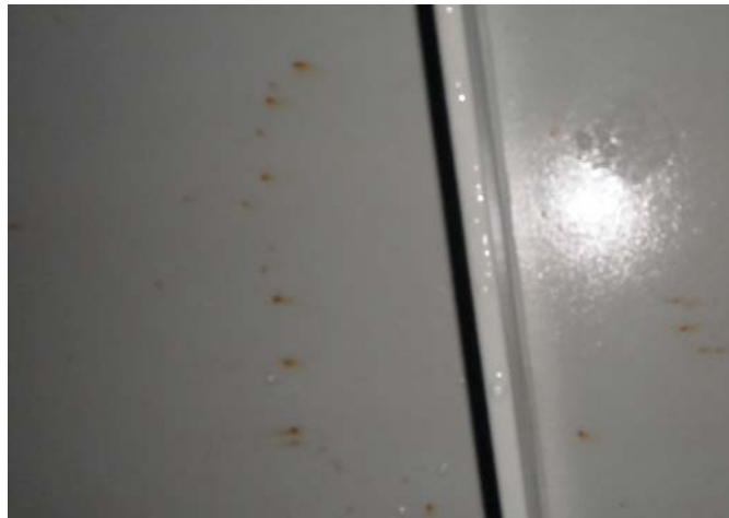
Picture 91 Pitting in the deckhead (Ask 2014c)
