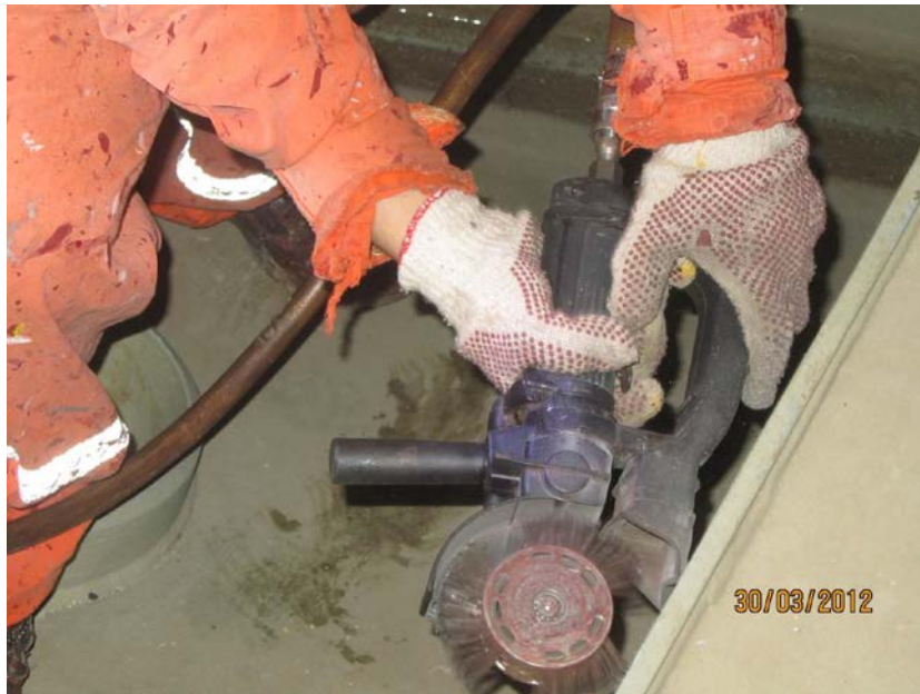
Picture 27 A bristle blaster used in the ballast tank (Solvang 2012)
