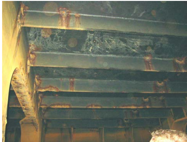
Picture 38 Coating in fair condition (IACS 2006)
