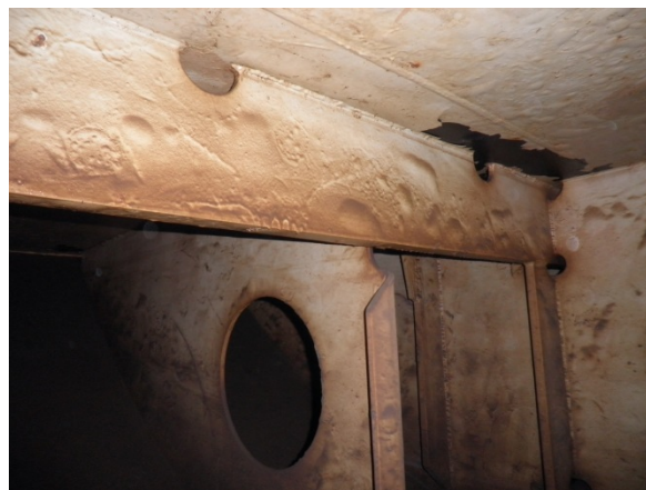
Picture 10 Large blisters in a double bottom ballast tank (Ask 2014a)
