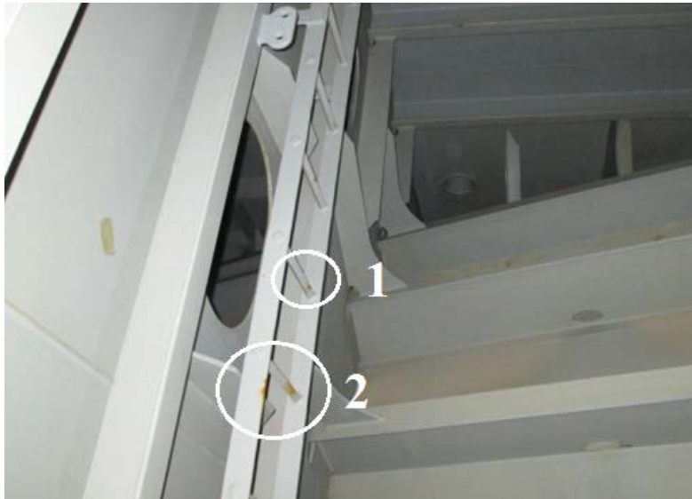
Picture 86 Ladder in fore peak tank (Clipper Posh 2014)
