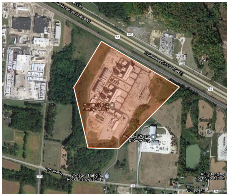
Figure 15-9: Hanging Rock Energy Facility in Ironton, Ohio. Covering a 20 hectares(0,2km) land plot (GoogleMaps, 2021)
