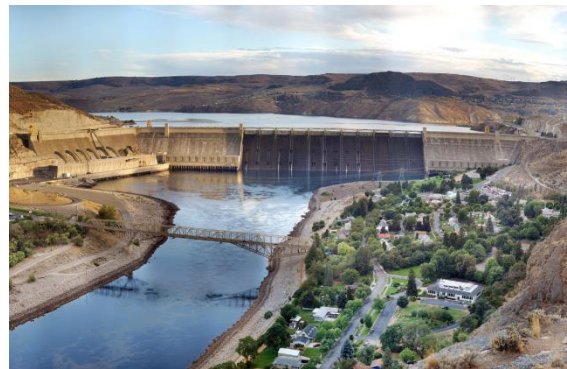
Figur 1-5: Grand Coulee Dam i staten Washington.
