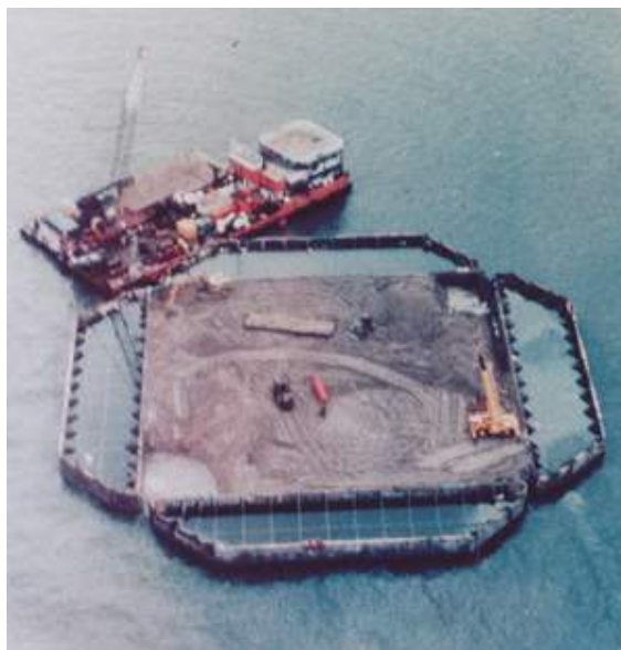
Figure 5.7: Tarsiut Island during construction (after Britner-Shen Consulting Engineers Inc.)
