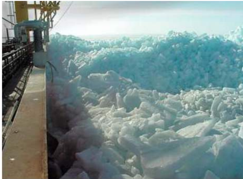
Figure 6.4 :Ice rubble built up in front of a wide structure in the Caspian Sea (Loset et al., 2006 with reference to Evers and Kühnlein, 2001).
