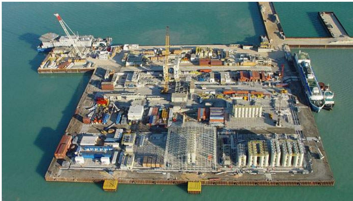
Figure 5.5: Sheet pile island built at the Kashagan field (Nymo, 2010).
