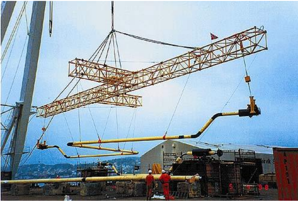
Figure 3-2 Horizontal spool lift (Stord Leirvik-Thaijournal.wordpress.com)
