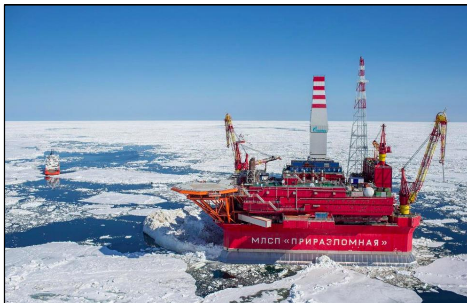
Figure 8 – Prirazlomnaya platform (Offshore energy Today.com, 2013)
