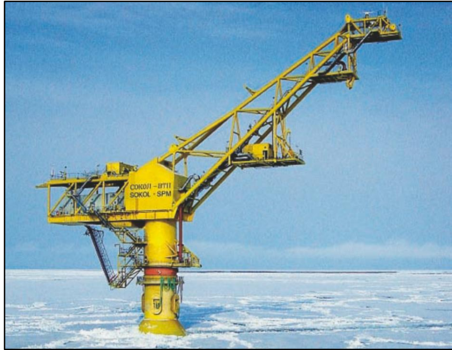
Figure 18 – Dekastri oil export terminal (Bluewater Company, 2009)
