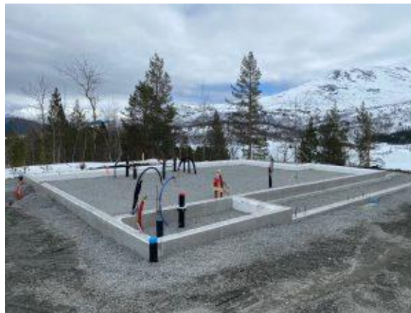
Figur 3.6.1 Stripefundament [27]
