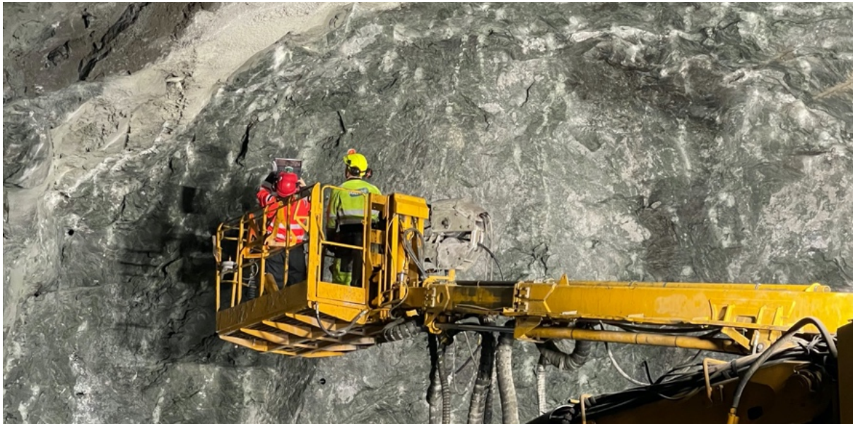
Figure 5: Photo showing safety attire and supervision and the required proximity to the rock wall face for using the terrestrial lidar scanner on the iPad Pro 2020 (Provided by A. Al-Samarray, 2022).
