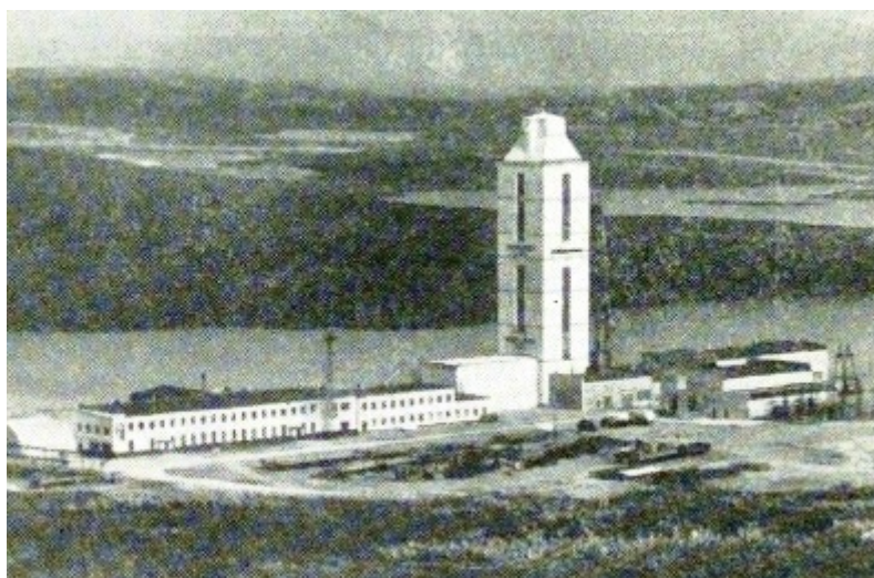
Fig.2 General view of Kola rig.
