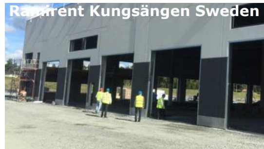
Precast Insulated wall panels of Kilenkrysset in Sweden. Both the weight and the thickness are reduced by 50%. [63]
