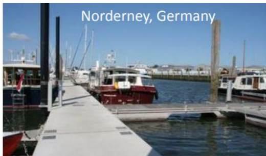
Pontoon in Norderney, Germany. It is corrosion free and 40% lighter than conventional reinforced concrete.
