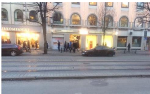
Road in Gothenburg, Sweden. MRC is used as the 20cm top layer of road surface at tram switching and signaling intersections.
