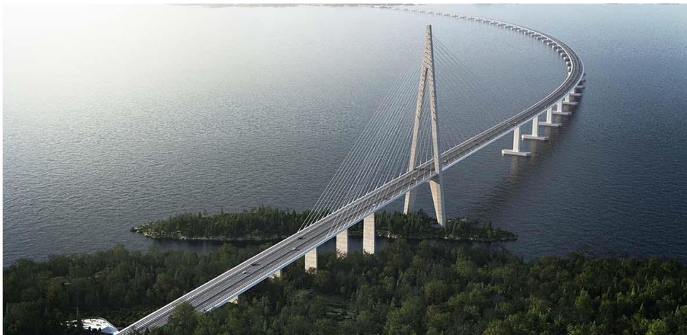
Figure 1-2: Proposed K12 floating bridge crossing of Bjørnafjorden [5]
