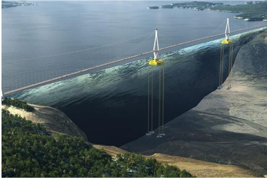
Figure 1-3: Section concept suspension bridge [6]
