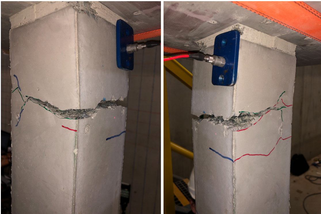
Figure 6.26. Major crack at Specimen10
