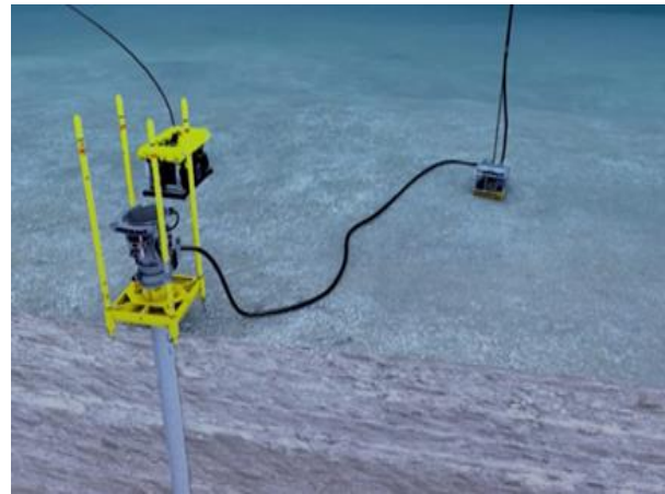
FIGURE 3: CLOSE-UP ON SUBSEA EQUIPMENT
