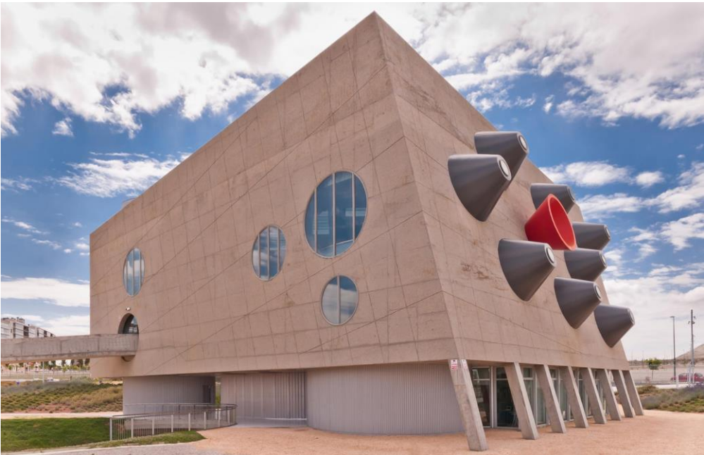
Figure 25. CUS building for the energy control and management (Valdespartera Ecodistrict, Zaragoza, n.d.)
