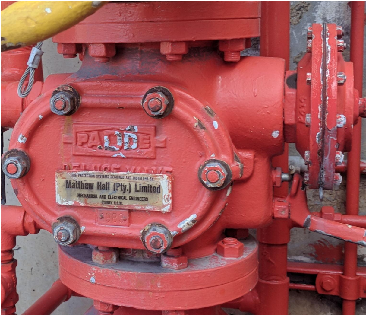
Figure 3: The original valve manufactured by PADDE, Wormald in 1983 [4]
