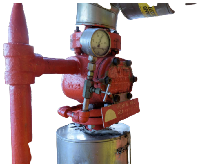
(b) Swing check valve configuration
