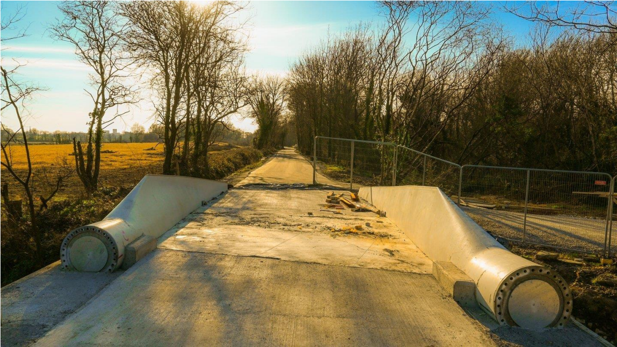
Figure A.8: BladeBridge constructed by the Re-Wind Network in Cork, Ireland. Photo by the Re-Wind Network (Deeney & Ruane, 2022).
