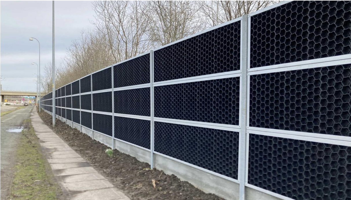
Figure B.3: Absorbent noise barriers made by Miljøskærm. Photo by Miljøskærm (Miljøskærm, 2021).
