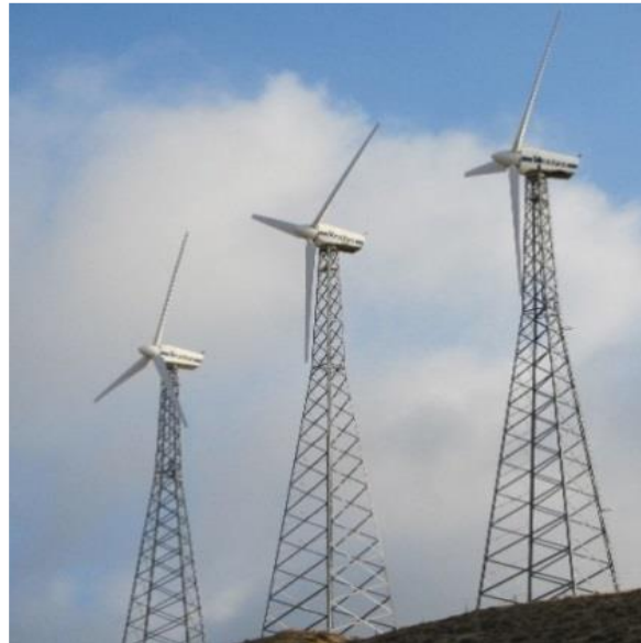
Figure 2 Lattice tower (Big Stone Renewables Services) (Saidur et al. , 2011)
