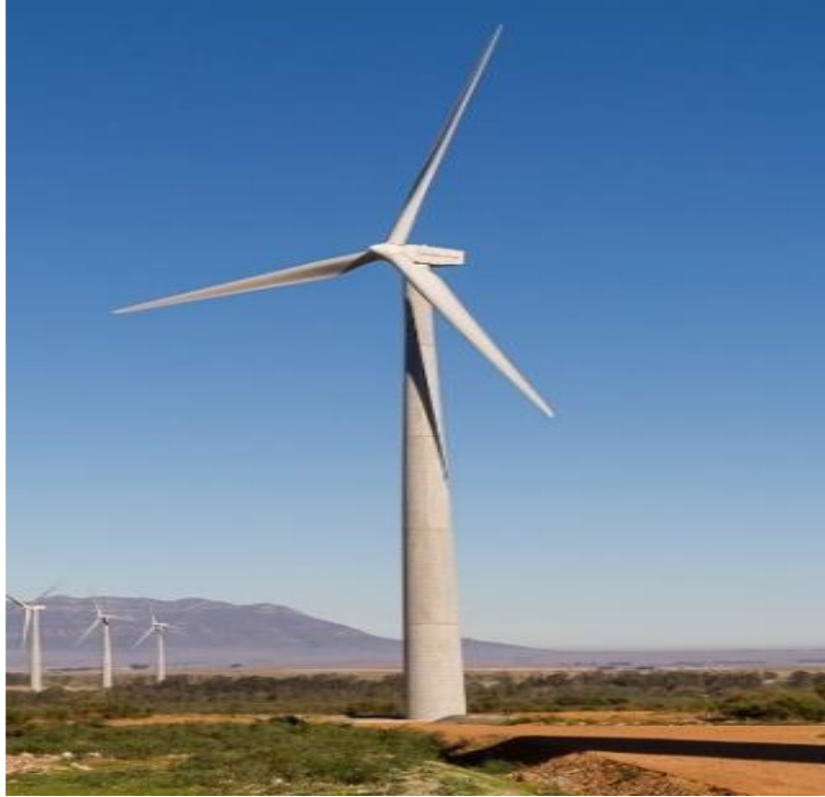
Figure 3 Concrete tower (Breton and Moe, 2009)
