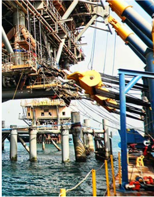
Figure 3 Illustration of the winches and wires, ref. [24]
