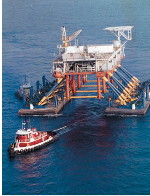
Figure 31 Illustrates the Versatruss system and the tug boats, ref. [37] (owner: Versatruss Americas; lift capacity 20,000 Te)
