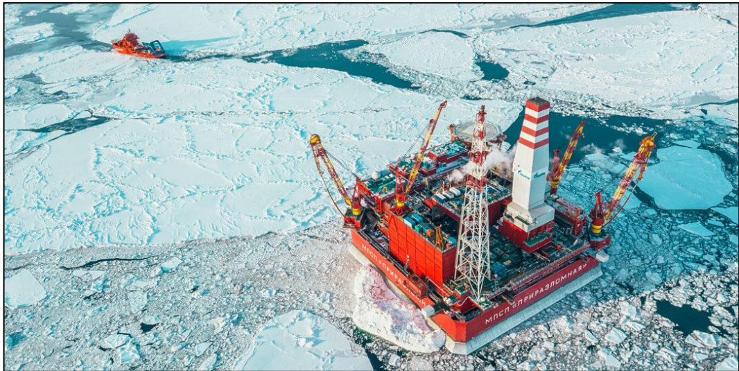
Figure 1.3 – Prirazlomnaya platform [s]
