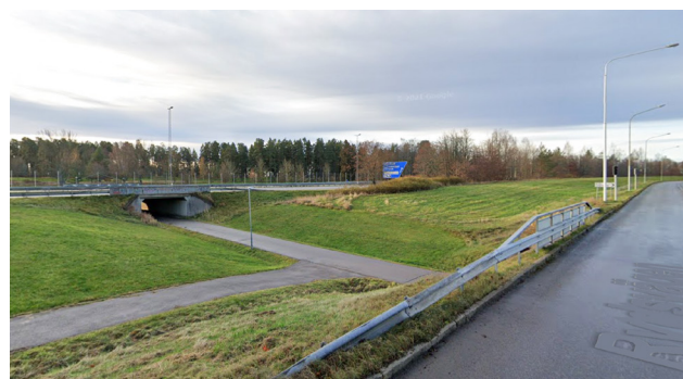
Fig. 41. Underground crossing on the route from Ryd (Google Maps, 2021)
