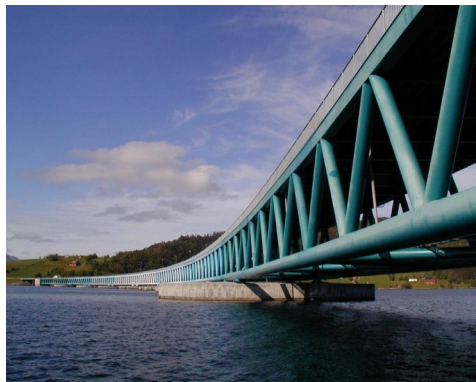
Fig. A.3 – Bergsøysund floating bridge. Opened in 1992.
