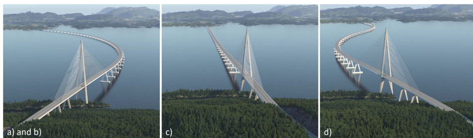
Fig. A.16 – Floating bridge sub-alternatives in 2019: a) curved bridge (without mooring lines); b) curved bridge with mooring lines; c) straight bridge; d) double-curved bridge.
