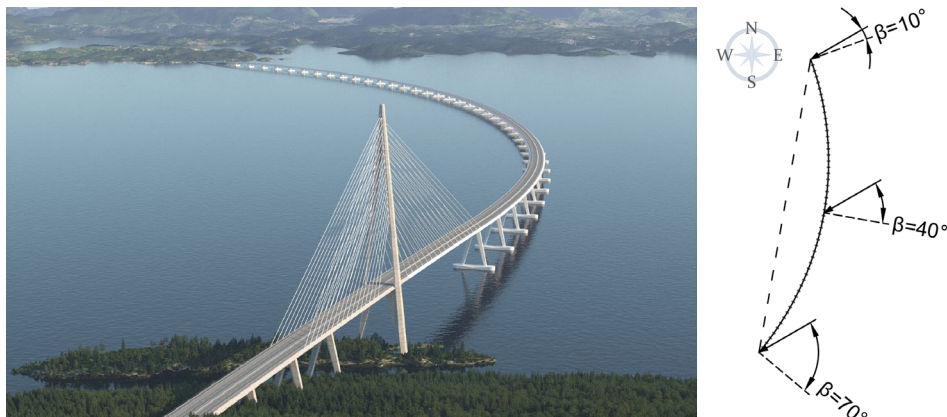
Fig. 6a – A planned floating bridge solution for Bjørnafjorden, Norway. Fig. 6b – Plan view sketch. Example of \beta variation for one mean wind direction.
