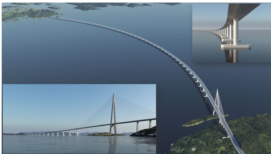
Fig. 11 – Illustration of the floating bridge alternative used as a case study (Norwegian Public Roads Administration, 2019a).
