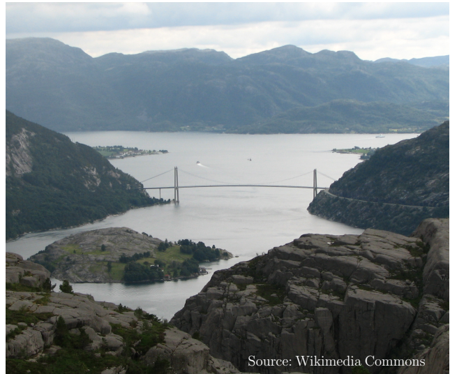
Fig. 1: East view of the Lysefjord Bridge site.
