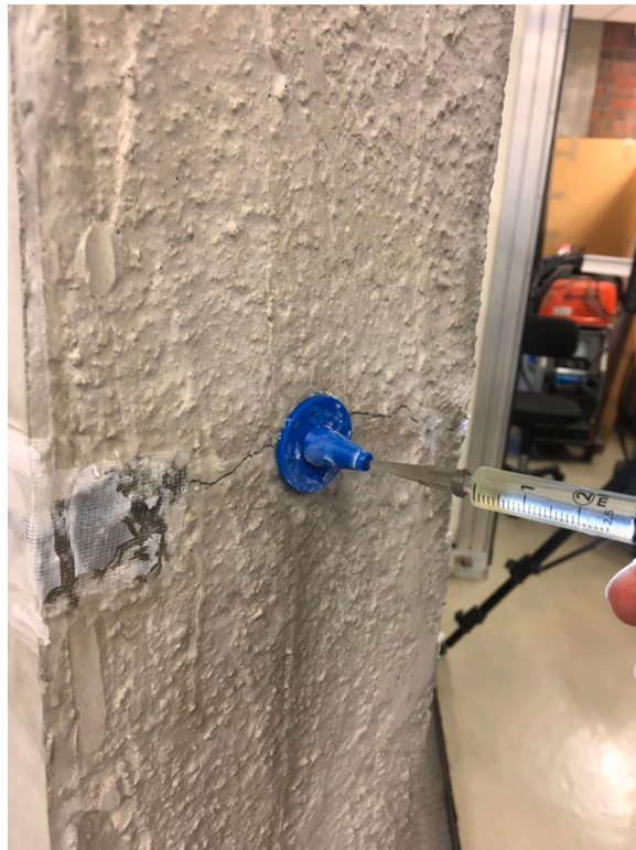
Fig. 4. Inserting the Mapepoxy BI-IMP to the crack through the surface packers.
