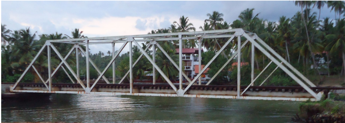
Figure 2. Considered railway bridge
