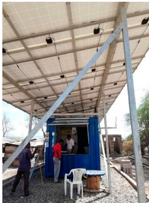
Figure 2. Mini-grid observed in Tanzania (Kitumbeine)
