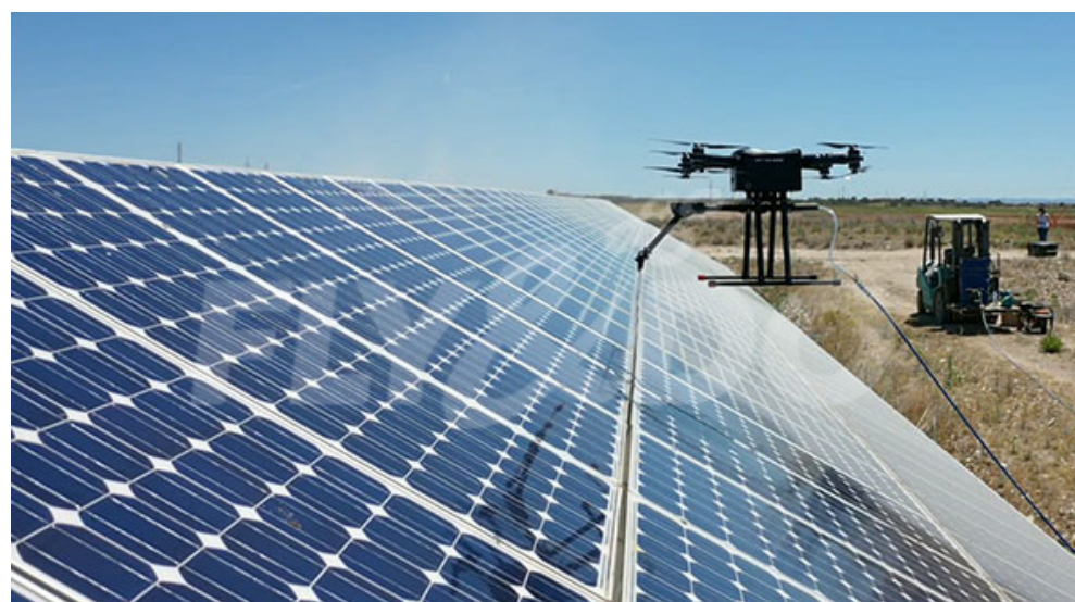
Figure 39. Drone-based PV cleaning [160].
