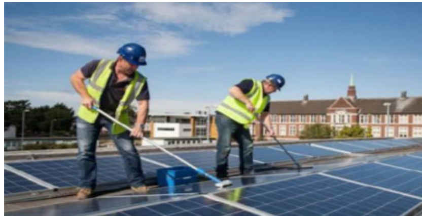
Figure 29. Manual cleaning of PV panels [135].
