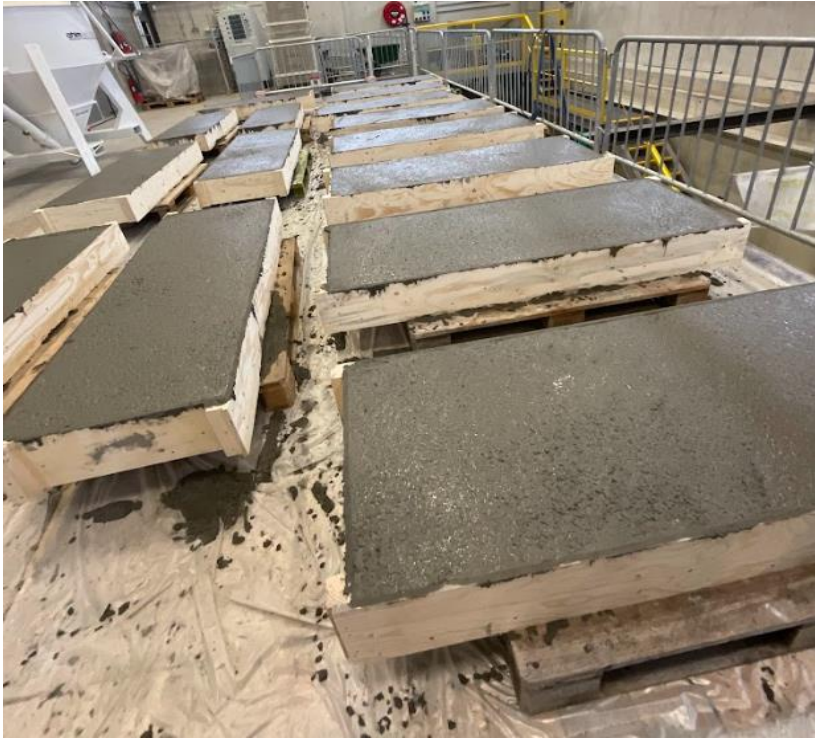
Figure 6.12 After concrete is poured
