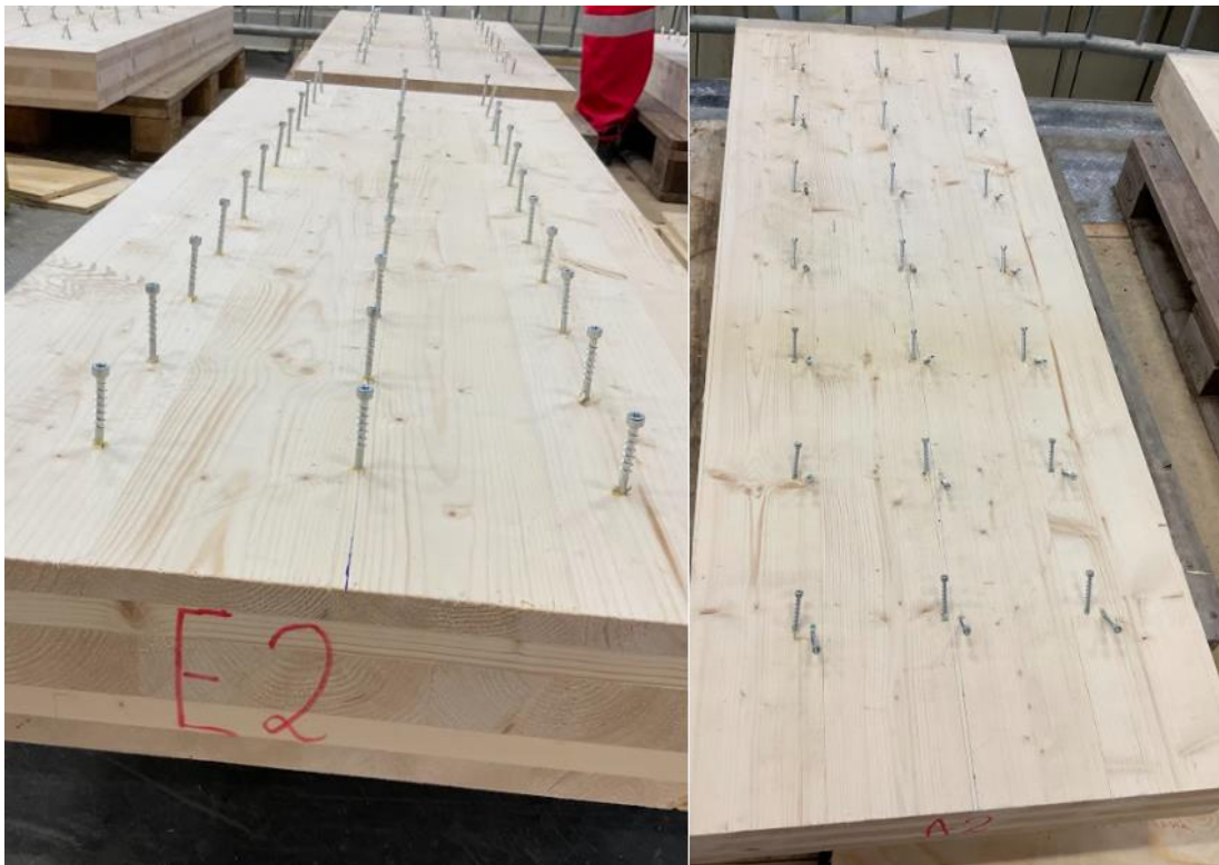
Figure 6.7 CTC installed in two different angles
