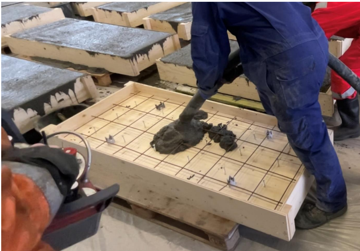
Figure 6.11 Pouring concrete
