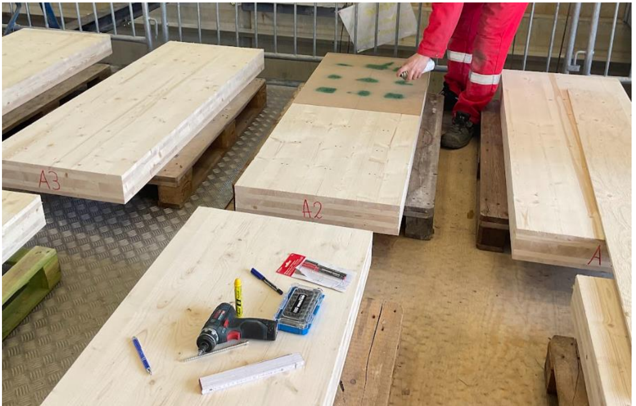
Figure 6.4 Preparing marks before installing screws
