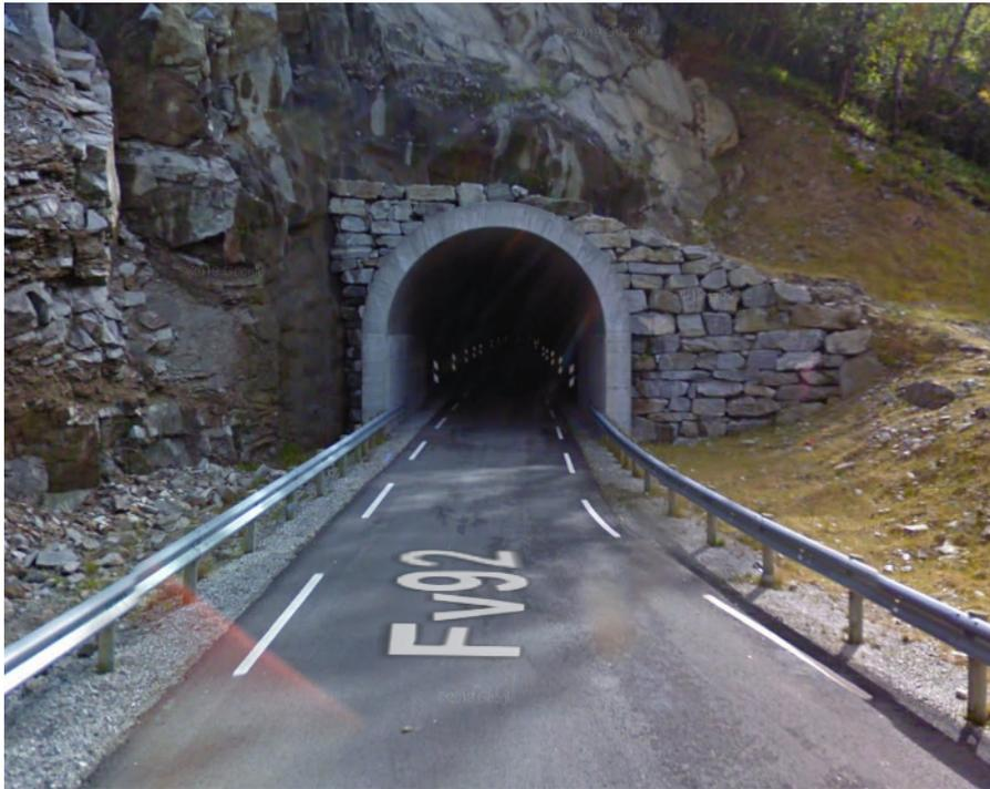
Figure 53: Dørefjelltunnelen with only one driving lane [8]
