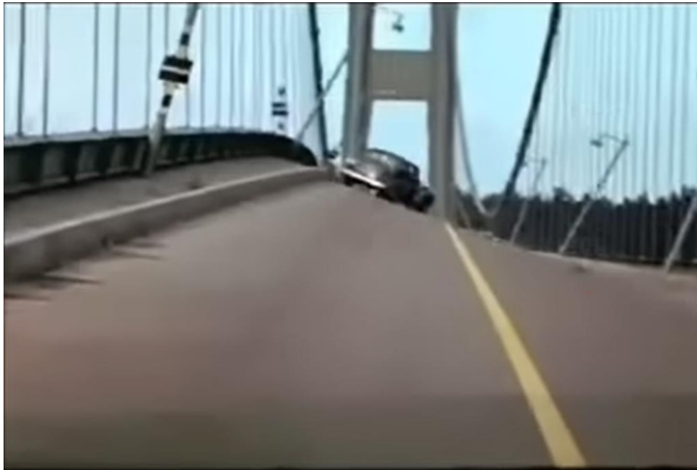
Figure 1: Tacoma Narrows Bridge as the wind induced destruction is imminent [1]
