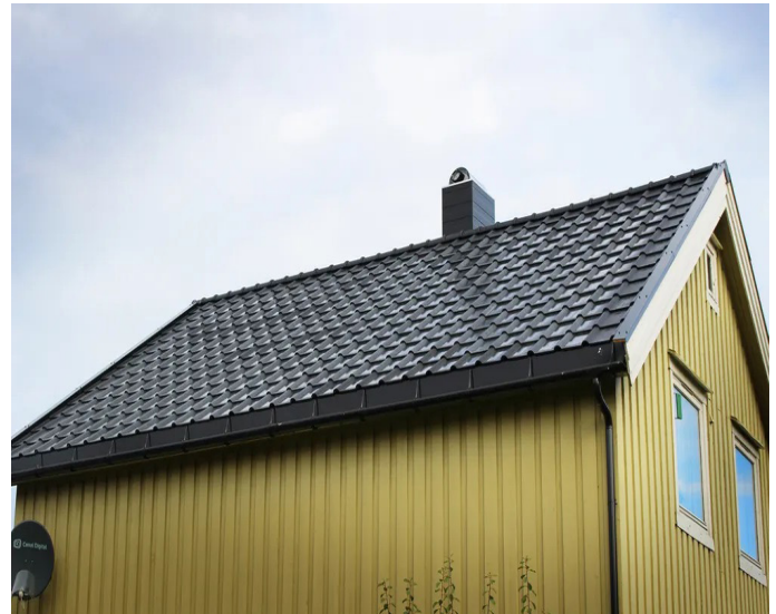
Figure 18: BIPV in roof tiles to give a realistic look on a tilted roof. Orkla Elektronikk. ( https://images.gfx.no/1000x563/1814/1814988/1200047361.jpg )
