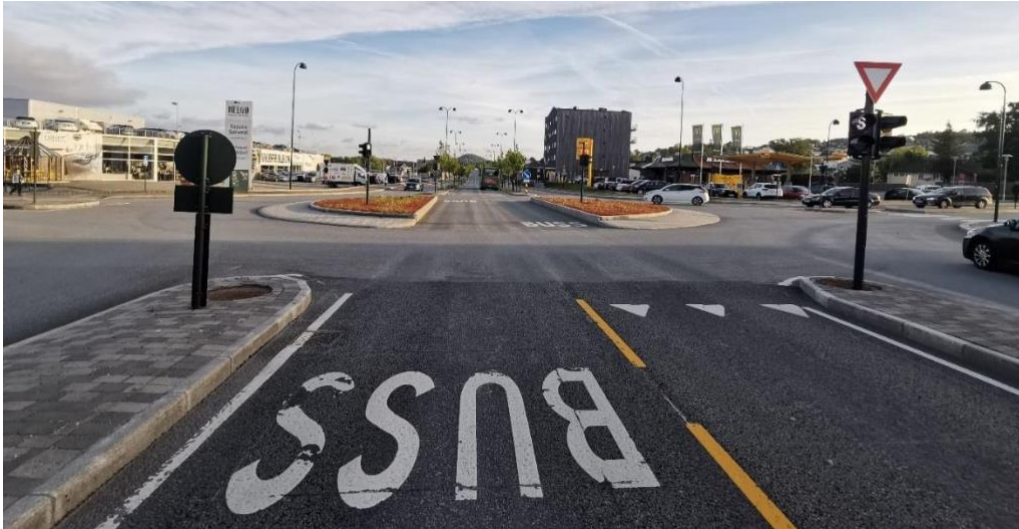
Figure 12 View on bus prioritized, signal-controlled roundabout in Mariero (authors picture)
