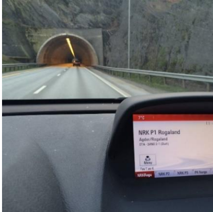
Figur 13 Radio bruk i tunnel (Gustavsen, 2016)
