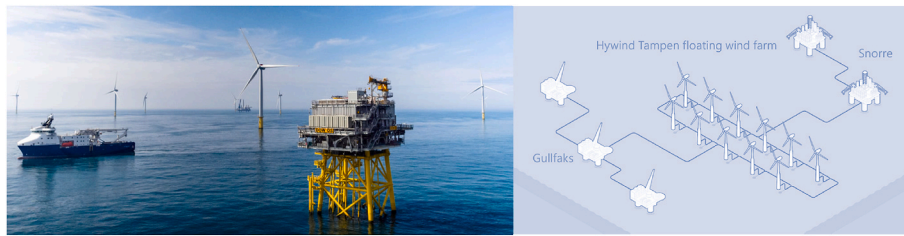
Fig. 1. The Hywind Tampen project and its connection to Gullfaks and Snorre fields (“Hywind Tampen approved by Norwegian”), (“Views from the industry”).
