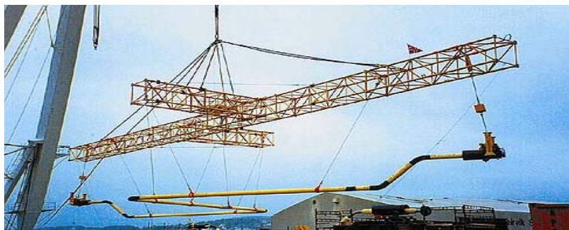
Figure 14: Spreader bars used for spool installation (Chan, Mylonas, & McKinnon, 2008)
