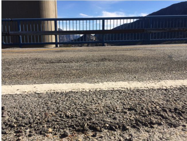
Figure 3.24: General pavement condition
