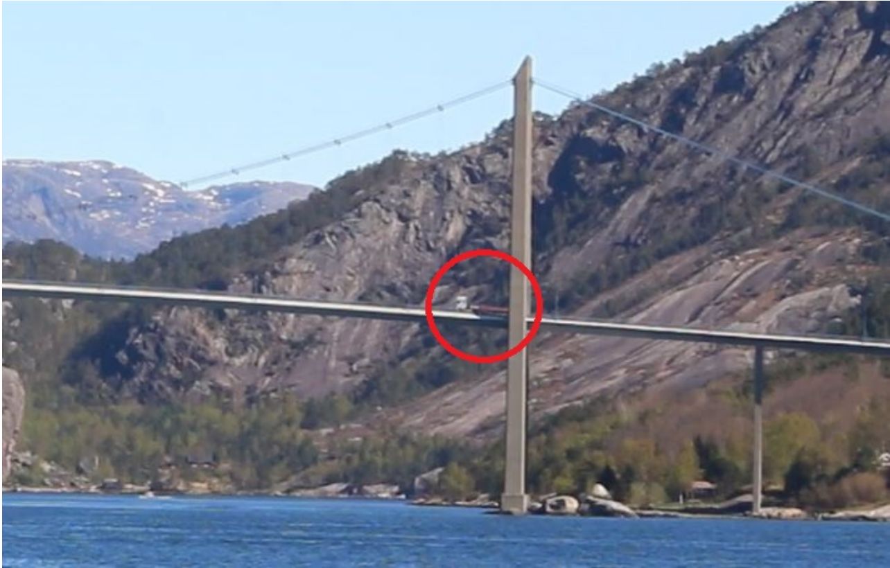
Figure 3.28: 50 tonnes truck entering bridge from the South at 23 km/h with a total cargo of 50 Tonnes
