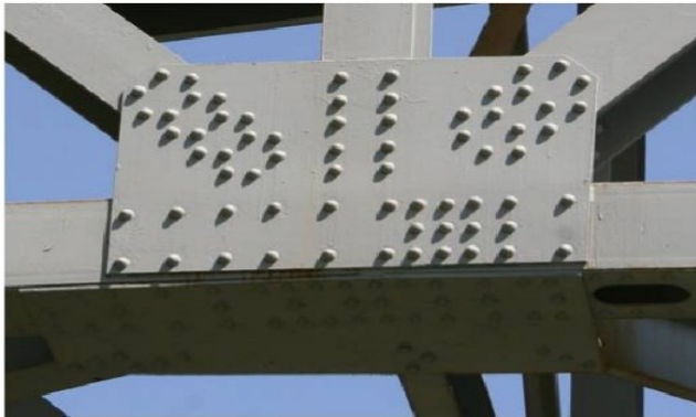
Figure 4: Gusset plate connection
