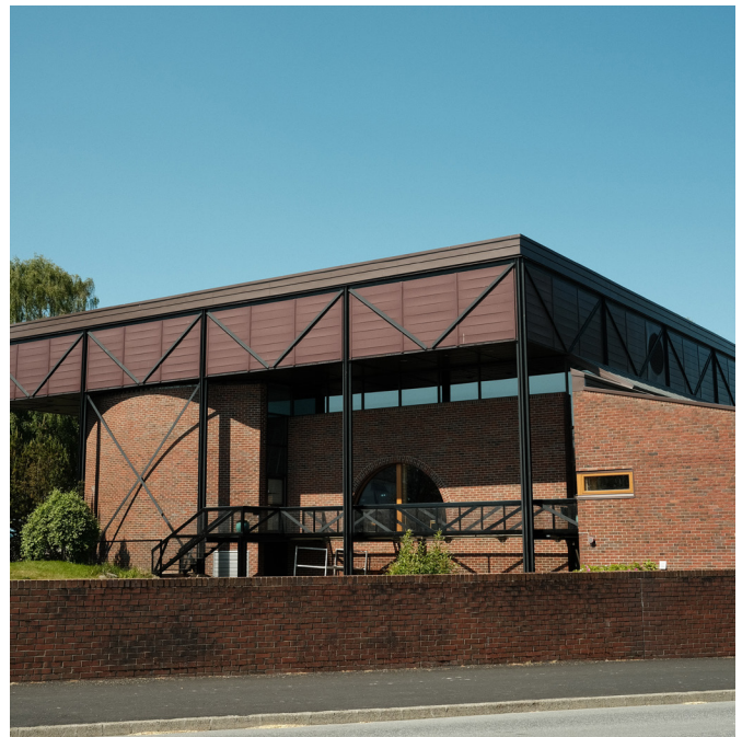
Figure 4.15: Picture of Bekkefare church
