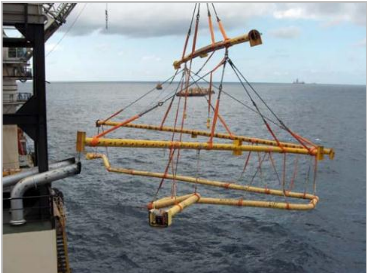
Figure 1-4 Spool lifting arrangement (Gloaguen, et al., 2007, p. 8)
