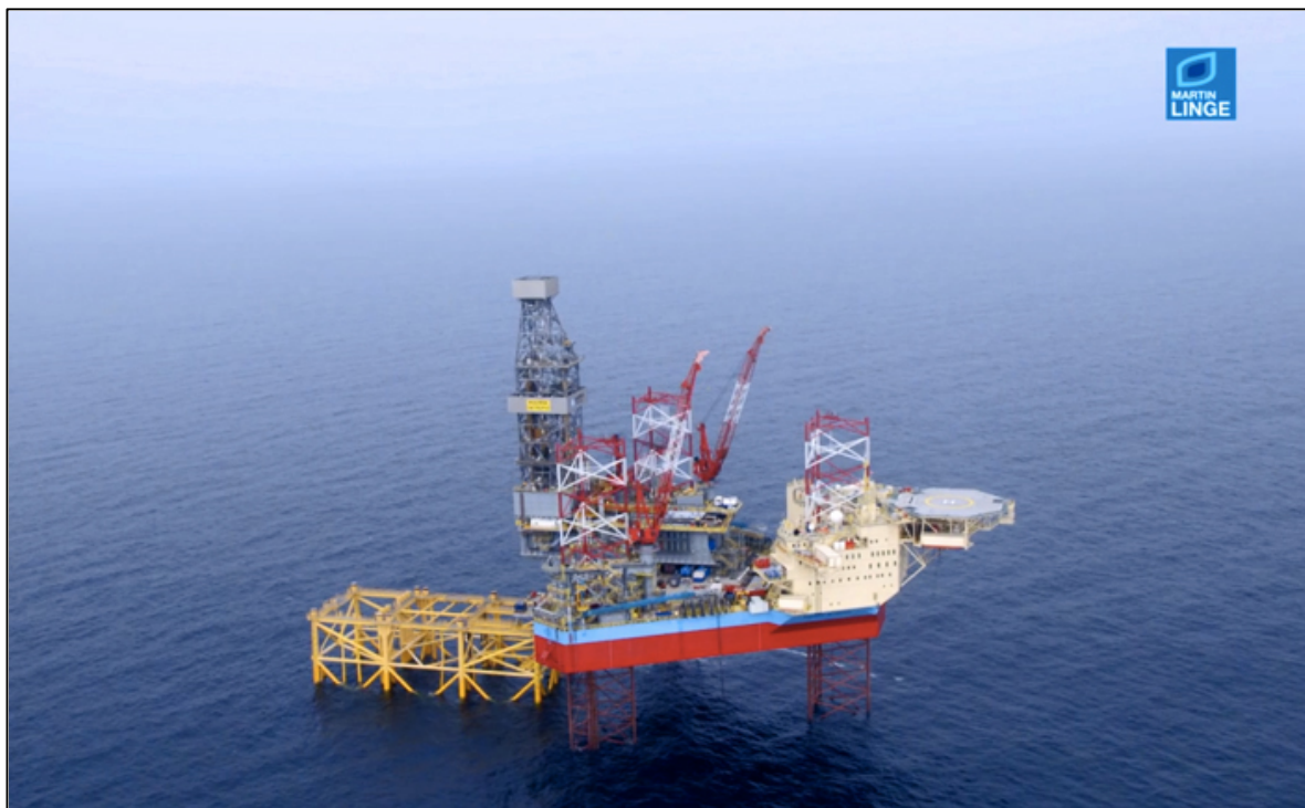
Figure 24: A jack-up drilling through a jacket substructure (32)
