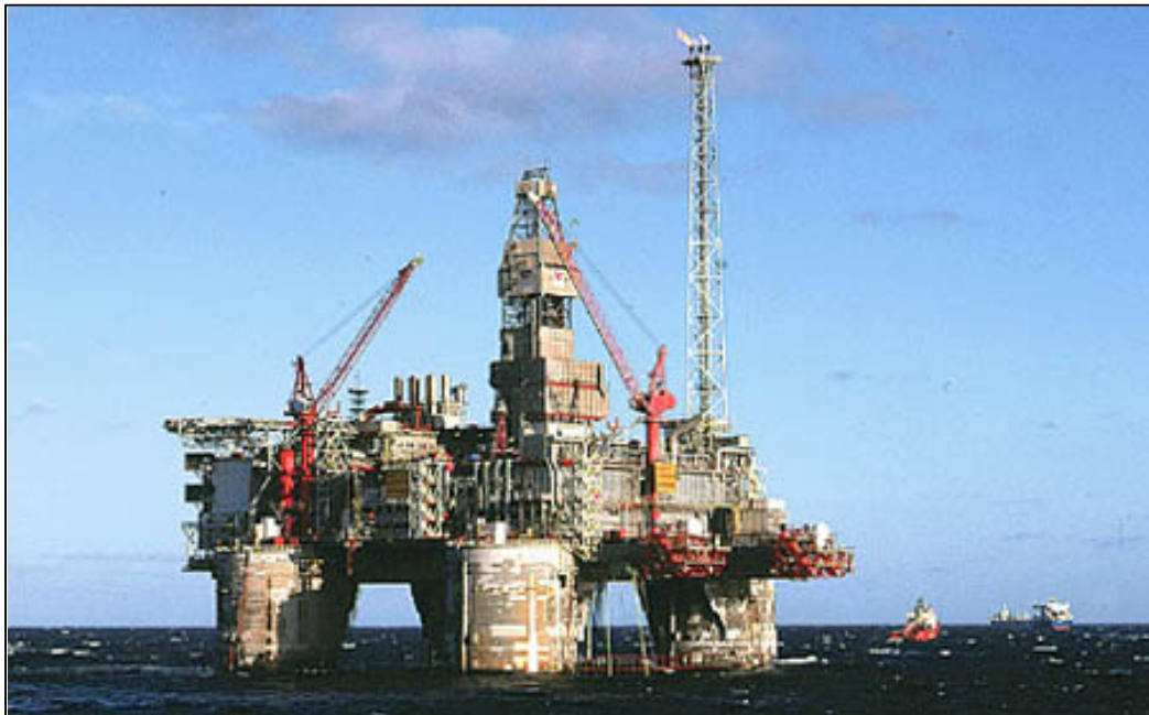
Figure 27: Heidrun concrete TLP (40)
