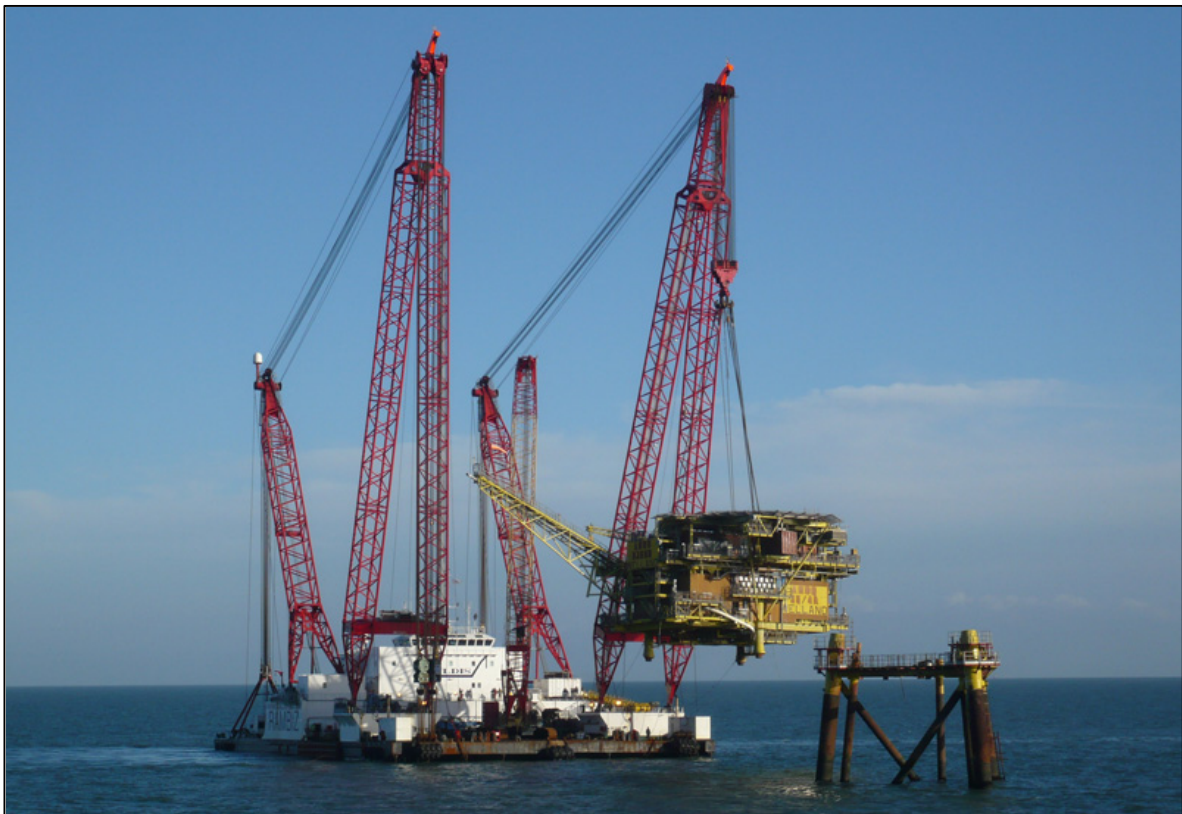
Figure 19: Decommissioning of a jacket platform (27)
