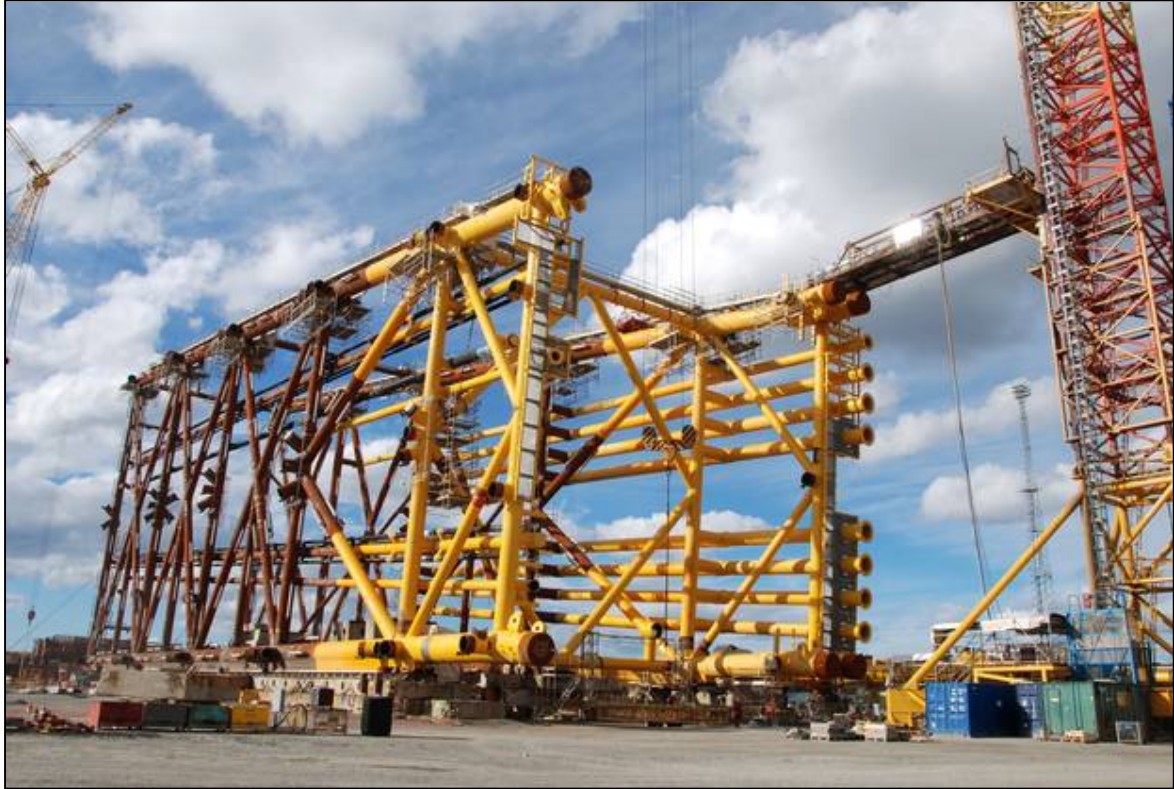
Figure 16: Construction of the Martin Linge jacket substructure in Verdal, Norway (22)
