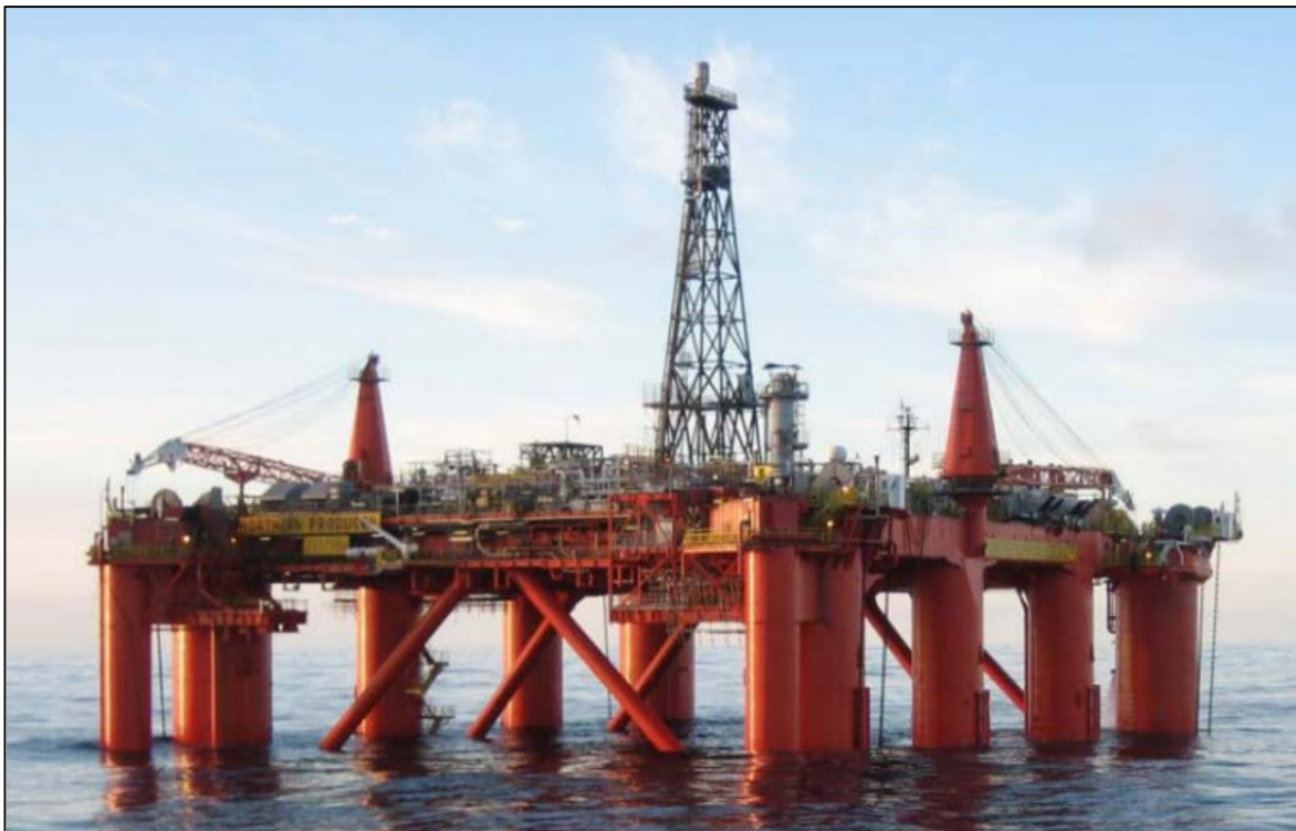
Figure 26: The semi-submersible platform Northern Producer (38)
