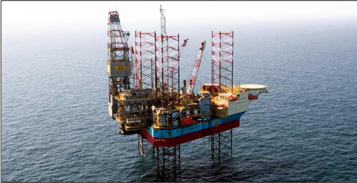
Figure 25: Volve jack-up drilling and production platform (36)
