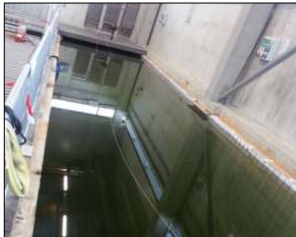
Figure 59: Tank filled with water
