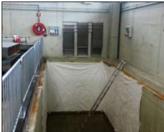
Figure 55: Process of covering the walls with the reflective material
