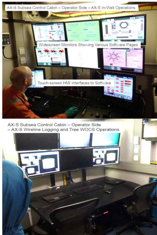
Figure 25: Subsea Intervention Cabin layout where the WOCS, wireline and other intervention operations are performed. The pictures were received from Expro to be used in this thesis.
